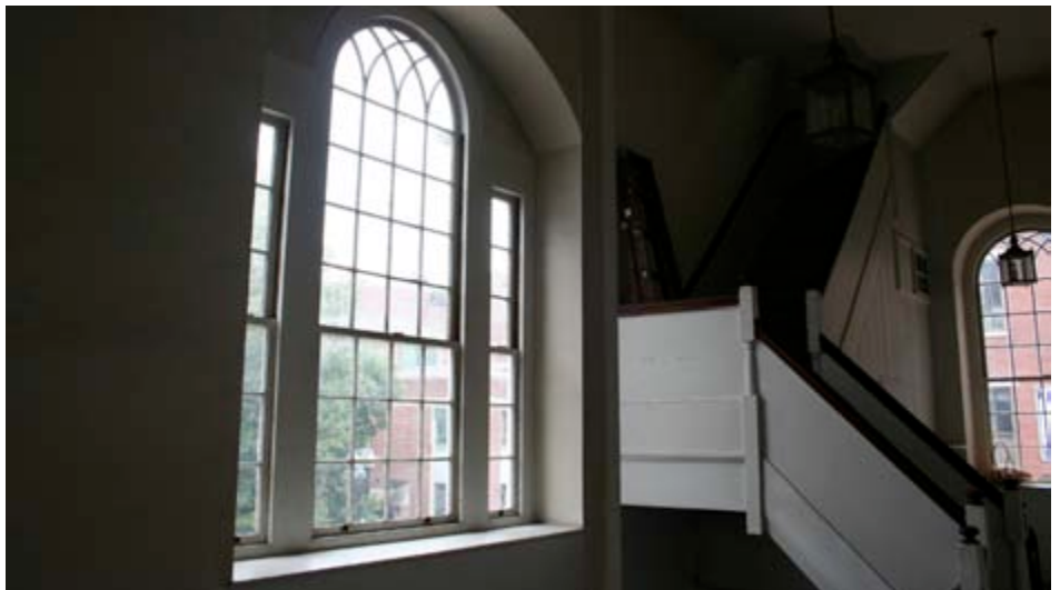
Palladian windows in the upper foyer with stairs leading to the bell tower.
