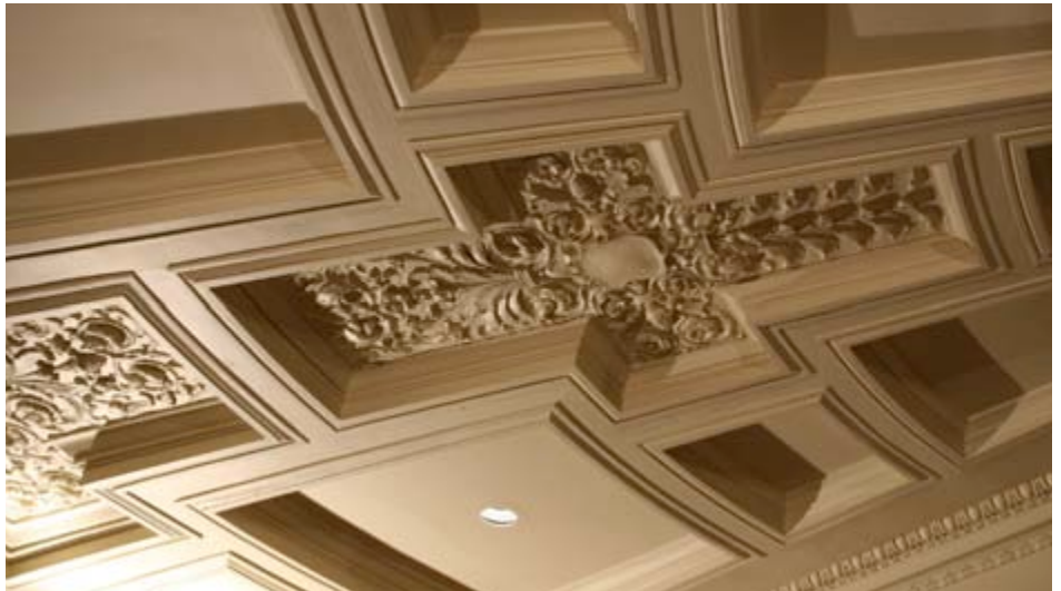
Cruciform coffers in the original lobby of the Extension building.
