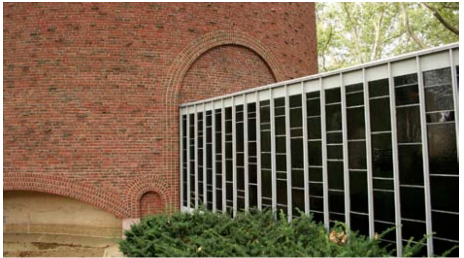
Brick arches, concrete foundation and moat meet the steel and glass entry passage.
