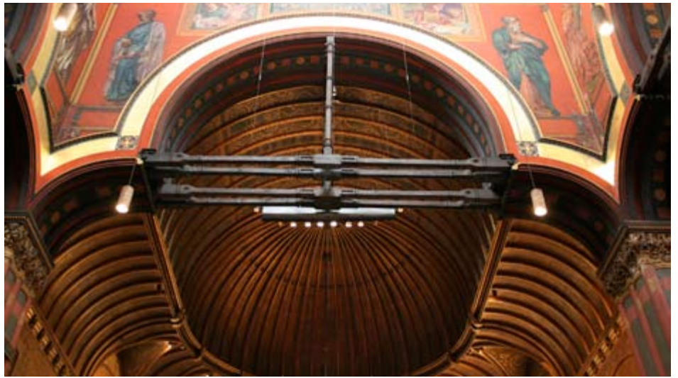
Structural ties secure the tripartite arches supporting the central tower and lantern above.
