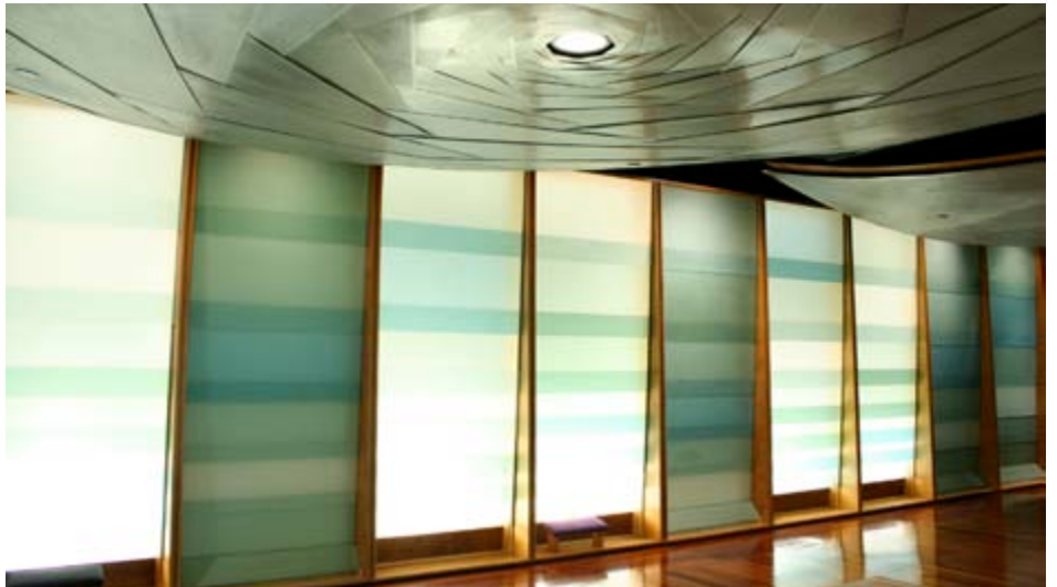
Back-lit layered safety glass casts a calming light into the space.
