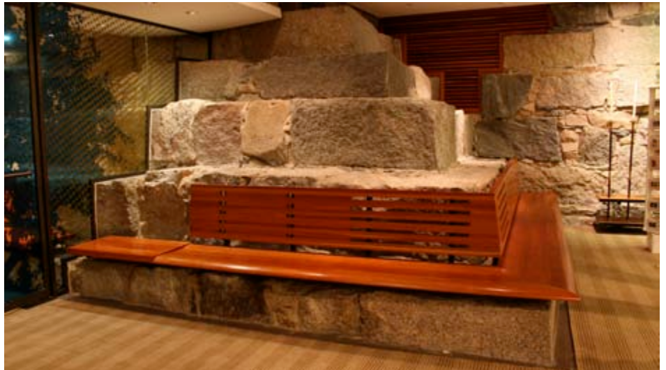
Pyramidal stone piers, integrated into the newly restored basement housing the gift shop.
